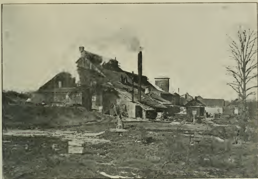
Canadian Goldfields, Limited ; arsenic refining plant.
