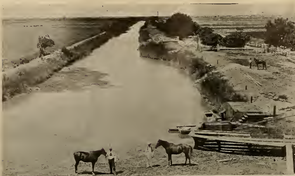
NAVIGABLE IRRIGATING CANAL.
