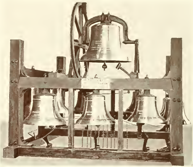
Chime of Twelve Bells, largest 4,300 lbs., as installed in the Tower of ST. PETER'S CATHEDRAL, Erie, Pa., 1903. Bell-Room 18 ft. Square by 16 ft. High.
