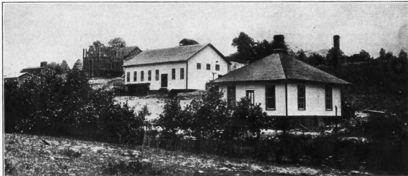
OFFICE AND MACHINE SHOP, KERSHAW MINING CO., KERSHAW, SOUTH CAROLINA
