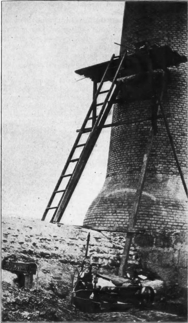
TESTING REVERBERATORY STACK GASES AT CIA. MINERA DE URURO, MACHAMARCA, BOLIVIA
