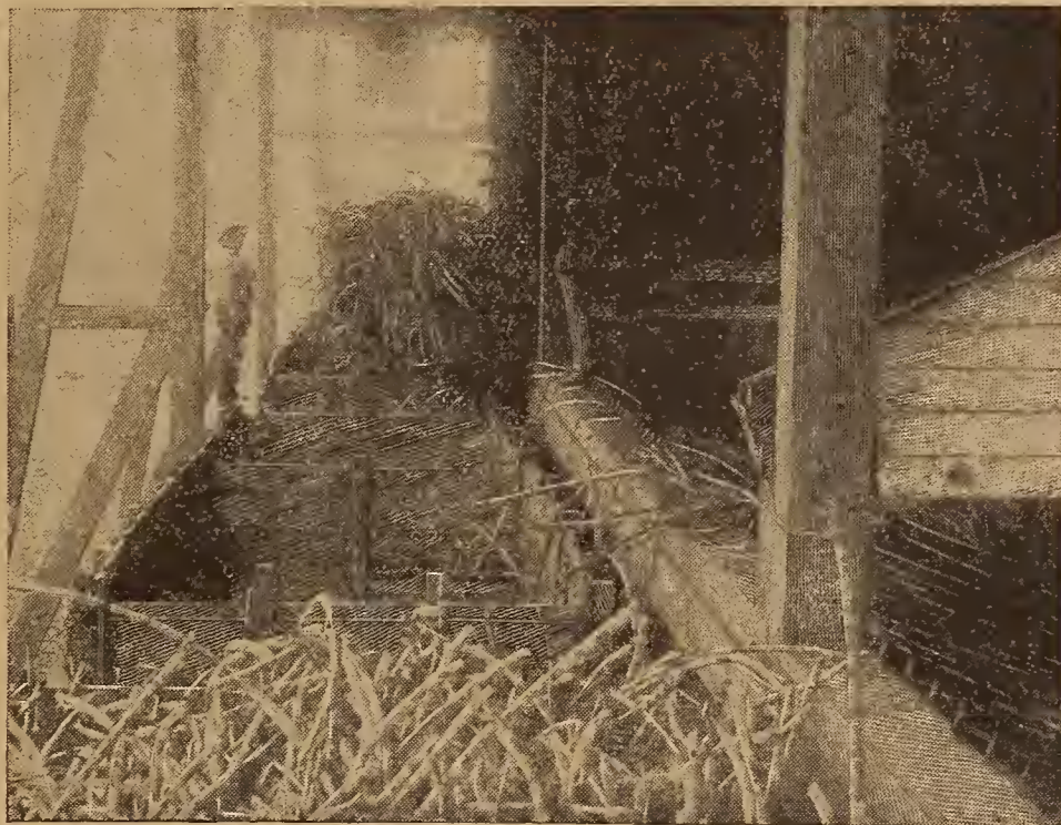
UNLOADING CARS WITH CHAIN SLINGS AT FACTORY.
