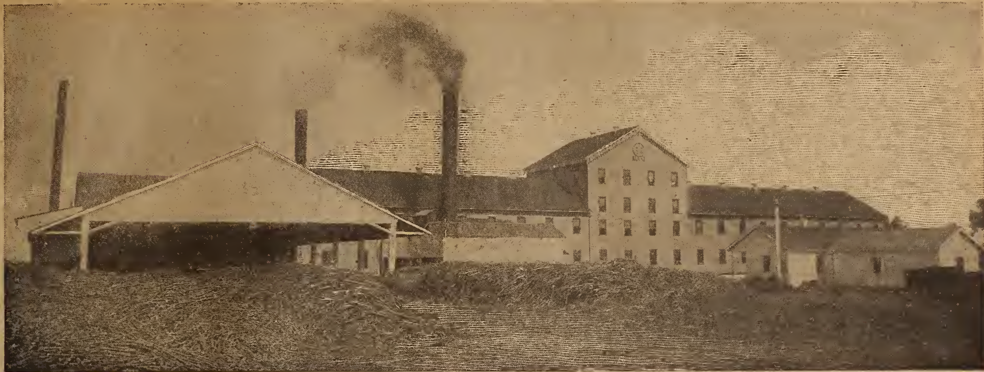
SUGAR-FACTORY AT SHADYSIDE PLANTATION, ST. MARY'S PARISH, LOUISIANA.
