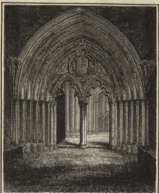
5th Entrance to the Charterhouse
