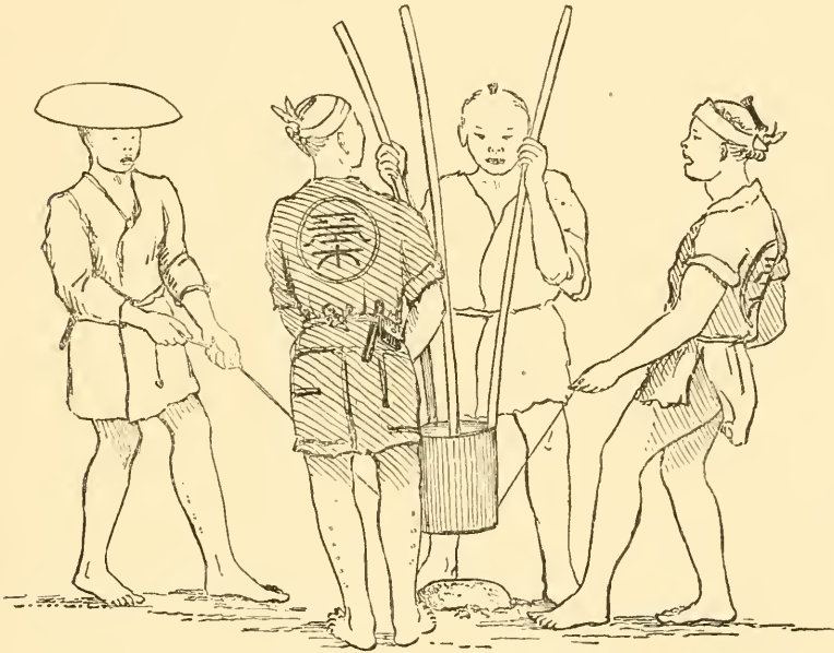
FIG. 5. — POUNDING DOWN FOUNDATION STONES.
