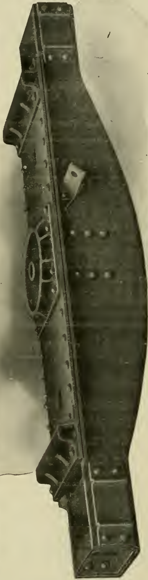
PRESSED STEEL BATH-TUB TYPE TRUCK BOLSTER.
