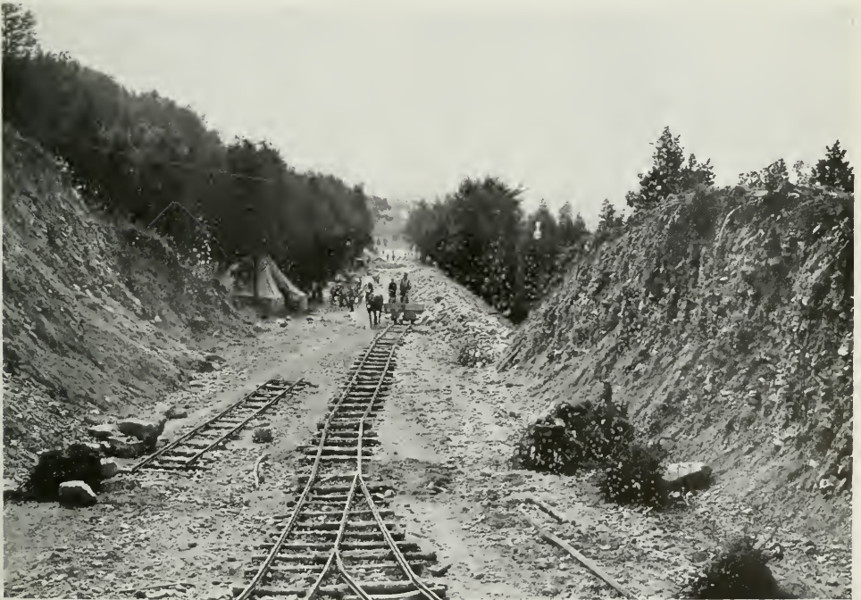
Niagara River Parkway North. Cut at Queenston Hill.
