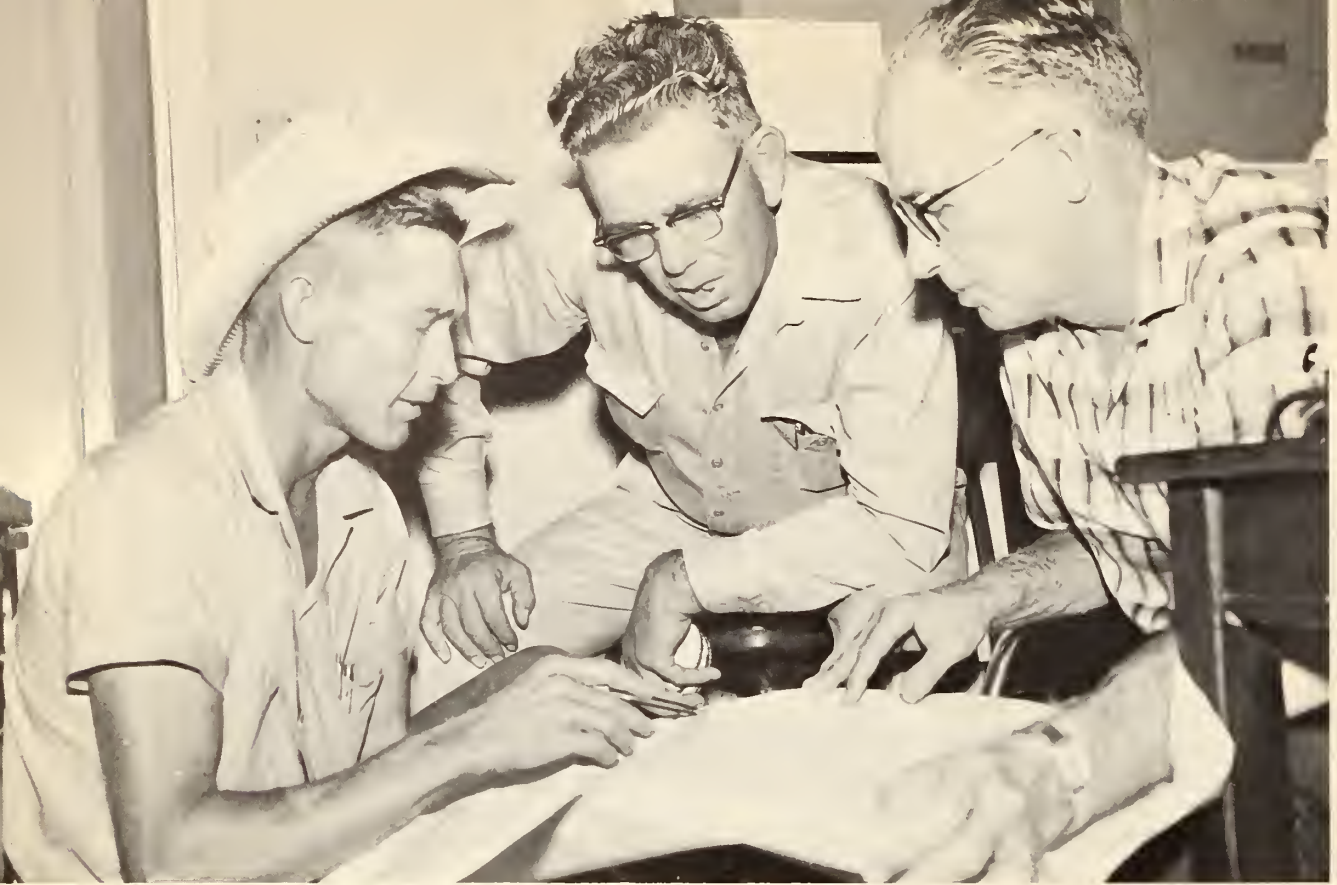
Co-op organizers worked closely with farmers and other rural people in choosing routes for power lines.
