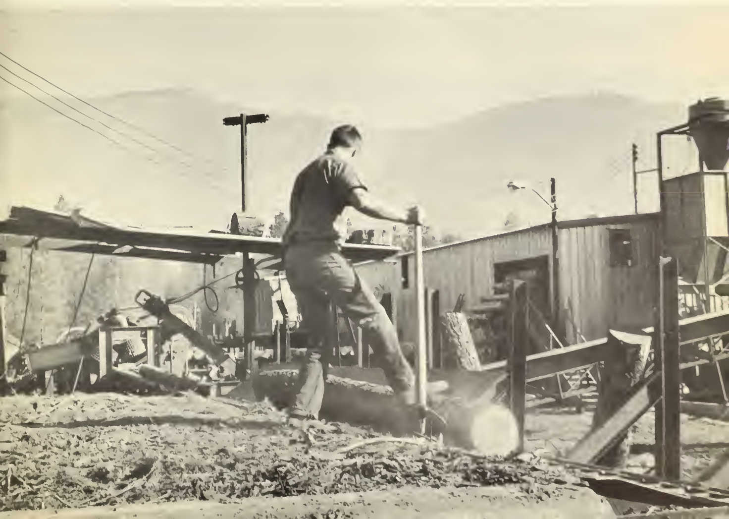
Removing bark from poles used to be a tedious operation before this electric debarker was installed.
