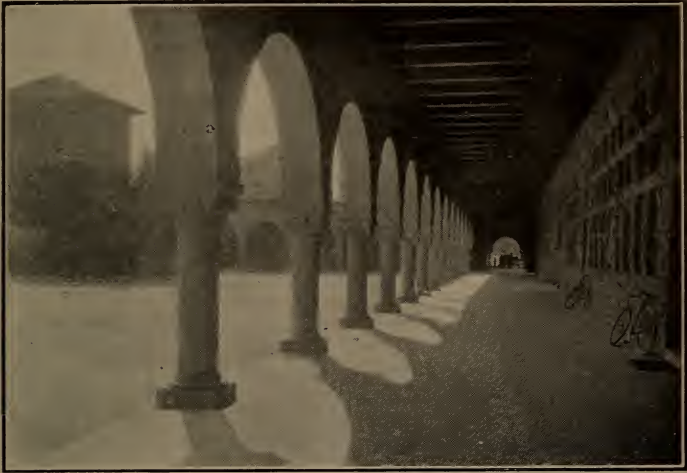
View of the Interior Court, Stanford University,
