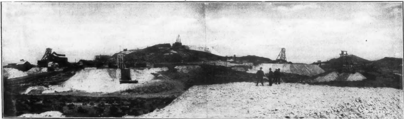
MINES AT GOLDFIELD. THE WHITE TALUS WAS, BEFORE ALTERATION BY VOLCANIC VAPORS, DARK-COLORED IGNEOUS ROCKS
