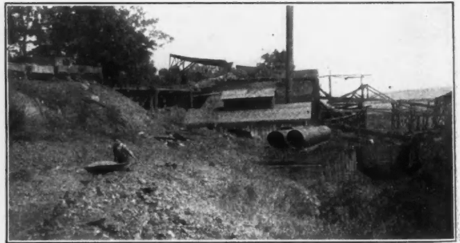
FIG. 5. NO. 3 LOG WASHER, IRONATON
