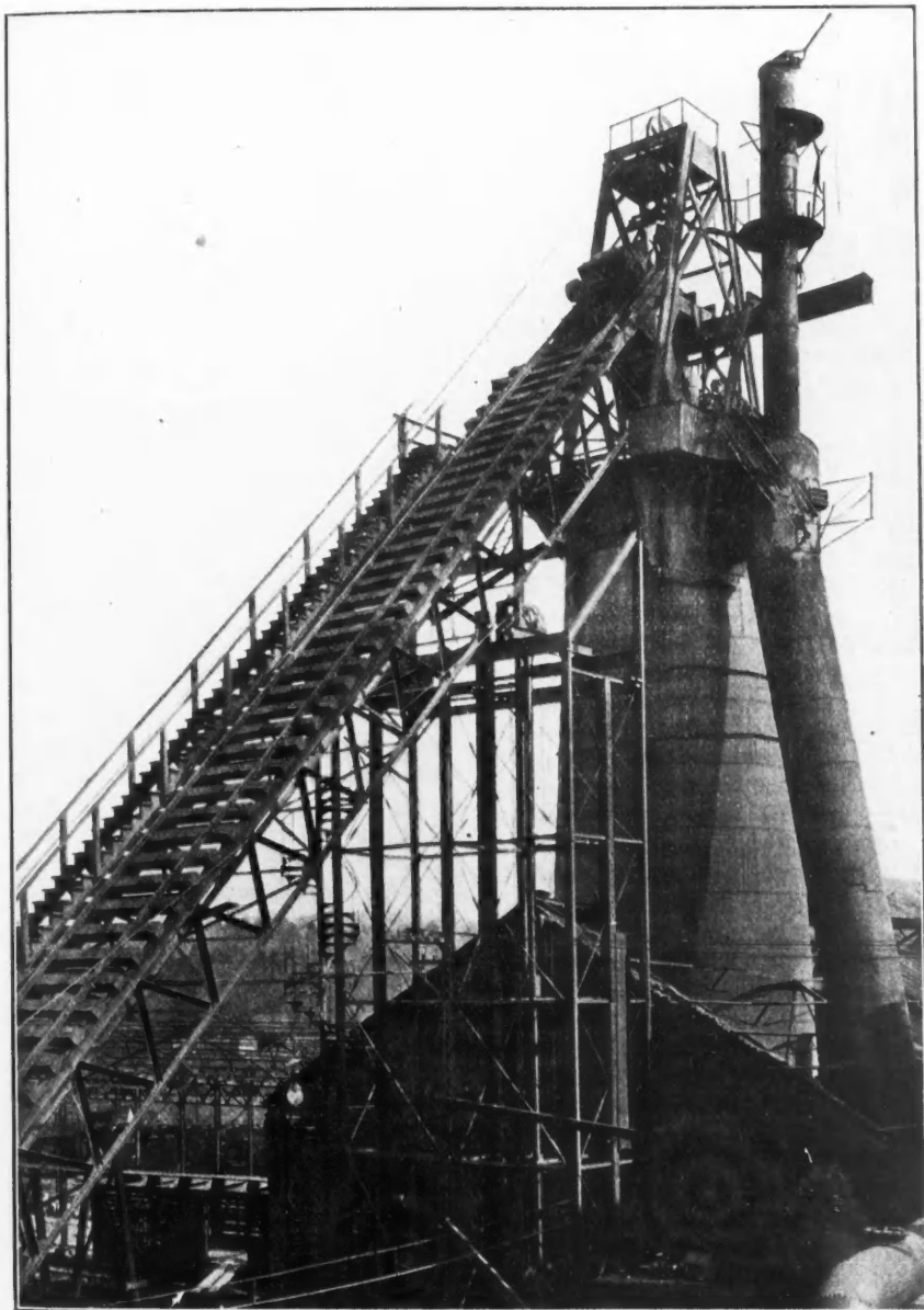
FIG. 9. NO. 1 FURNACE, IRONATON, SHOWING BAKER TOP
