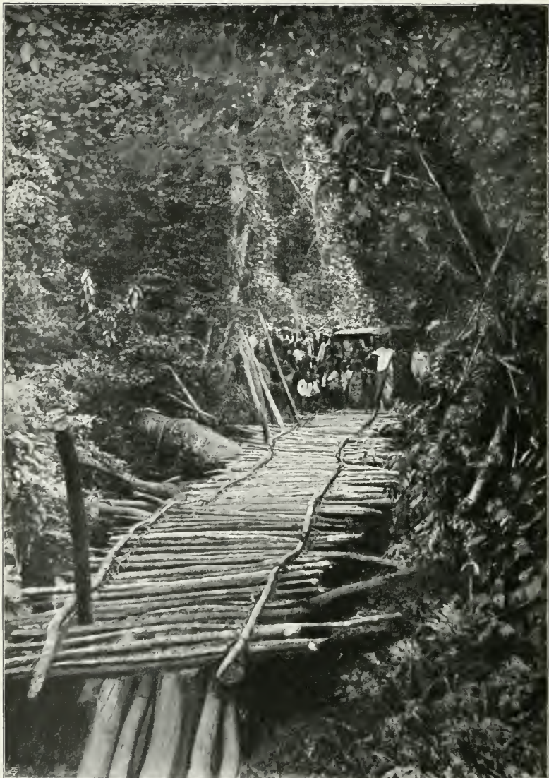
Fig. 5.—NATIVE STICK BRIDGE. Weak and insecure.
