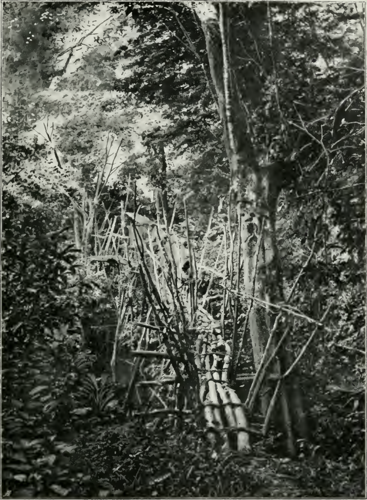
Fig. 6.—A HIGH TRESTLE BRIDGE OVER DEEP RUNNING STREAM. SHERBRO DISTRICT.
