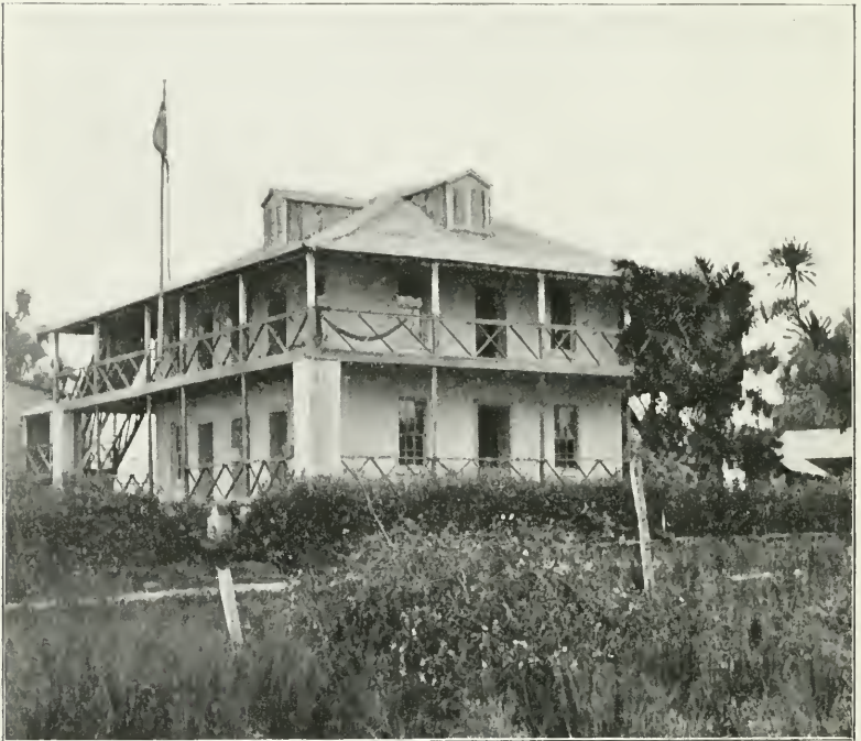
Fig. 8.—GOVERNMENT HOUSE, BONTHE, The Residence of the District Commissioner.
