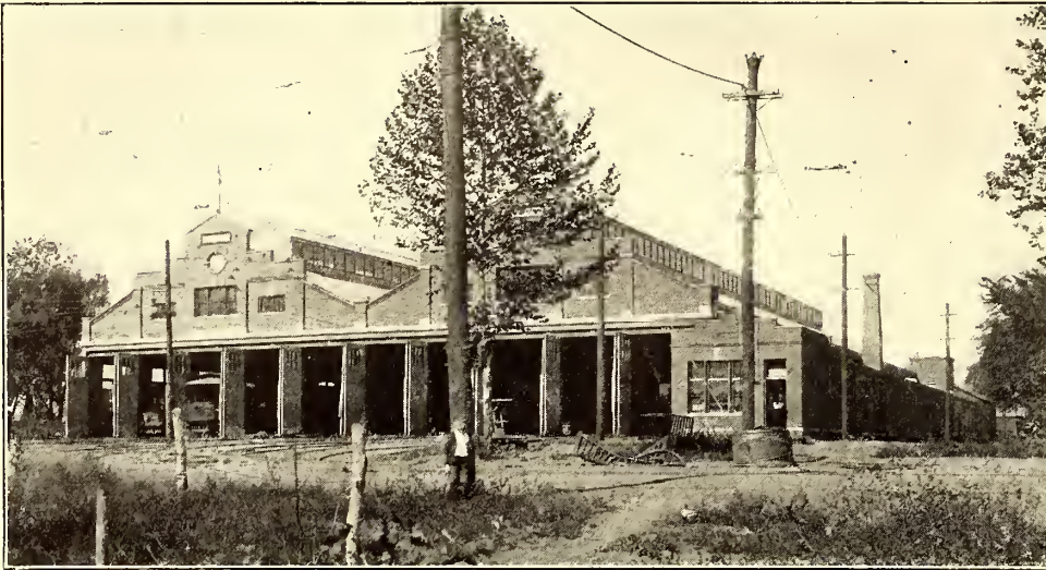
THE REPAIR SHOP AND CAR HOUSE AT NEWARK
