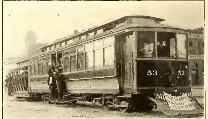
MOTOR CAR WITH OPEN TRAILER AT DENVER
