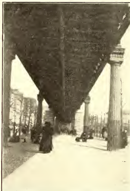
VIADUCT ON A BOULEVARD
