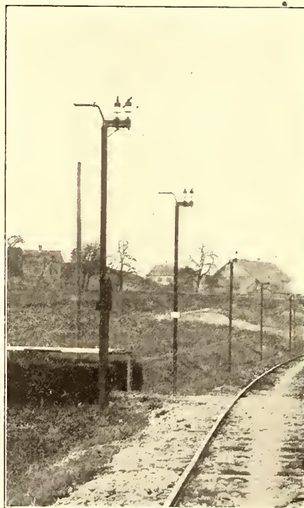
FIG. 6.—ARRANGEMENT OF THE CONTACT LINE AT AN ORDINARY CROSSING
