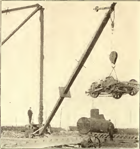
MOTOR-DRIVEN DERRICK LIFTING CAR TRUCK
