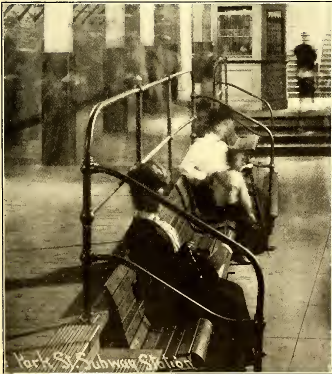
FIG. 5.—PHOTOGRAPH USED TO PROVE STATION STAIRWAYS WERE AMPLY GUARDED BY RAILINGS
