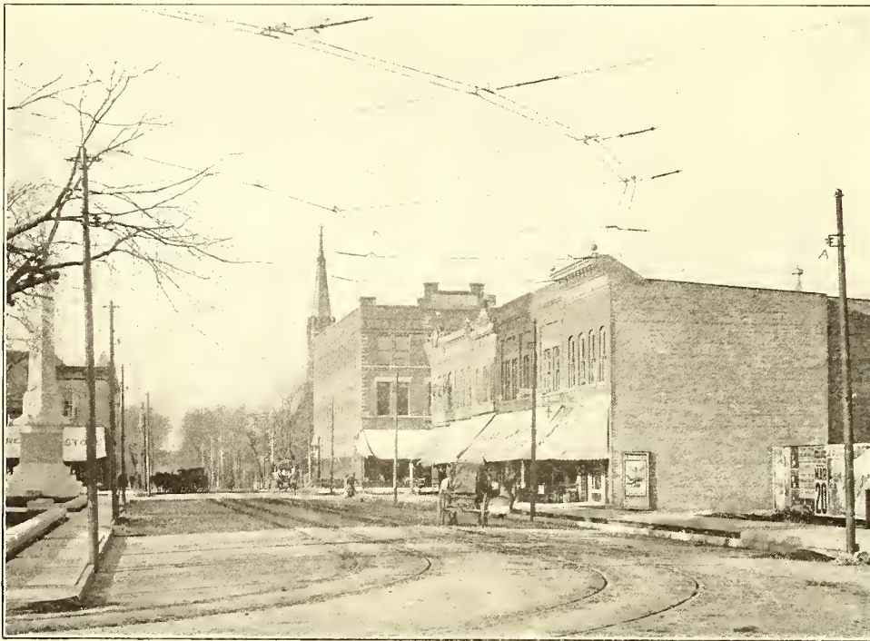
FIG. 14.—VIEW OF OVERHEAD CONSTRUCTION IN PONTIAC
