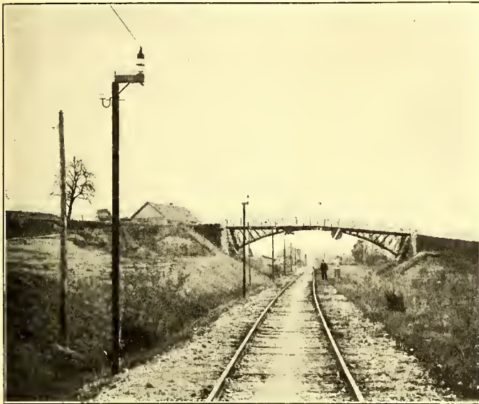
FIG. 9.—ILLUSTRATING AN INSTANCE WHERE A GOOD BRIDGE CLEARANCE MAKES UNNECESSARY THE SHIFTING OF THE CURRENT COLLECTOR PIVOT
