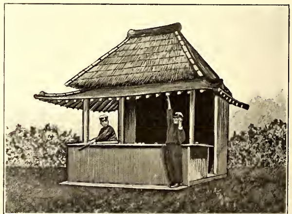
ONE OF THE JAPANESE BUILDINGS UNDER CONSTRUCTION
