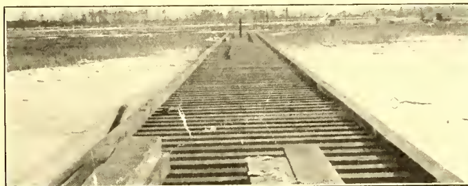
TRESTLE BUILT WITH PORTABLE PILE DRIVER
