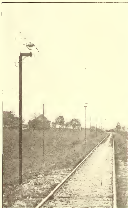
FIG. 5.—ANOTHER VIEW OF THE "INVERTED" CATENARY SUSPENSION
