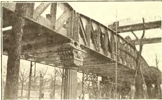
STANDARD VIADUCT DURING ERECTION, PARIS METROPOLITAN RAILWAY
