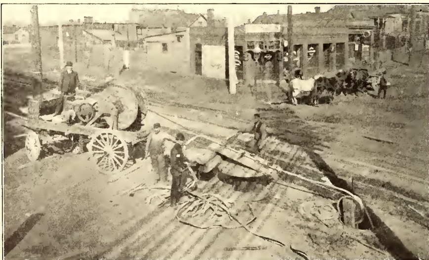
FIG. 2.—STRIPPING LEAD-COVERED CABLE AT ST. LOUIS
