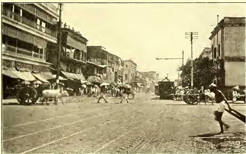
VIEW AT THE INTERSECTION OF THE HONRAH BRIDGE APPROACH
