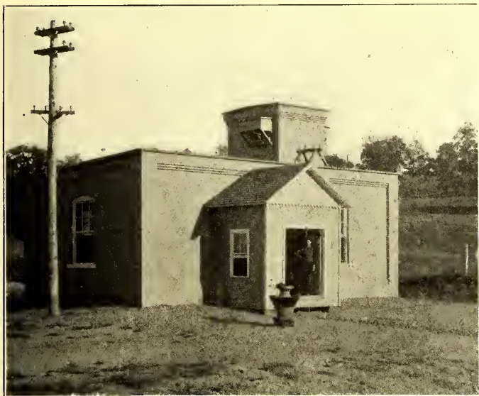
THE PLEASANT VALLEY SUB-STATION
