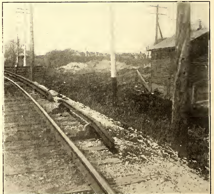
AUXILIARY RAIL LAID FOR ALARM CIRCUIT
