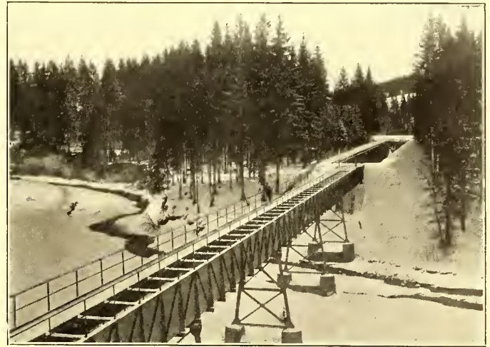
MILL RACE CROSSING THE RIVER AMMER BELOW INTAKE, BY MEANS OF STEEL AQUEDUCT
