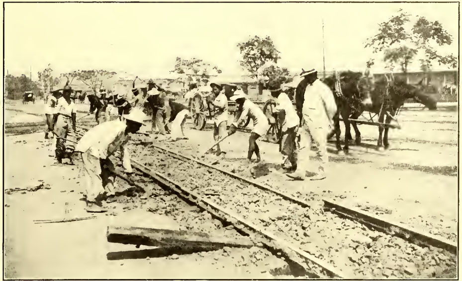
TEARING UP OLD T-RAIL
