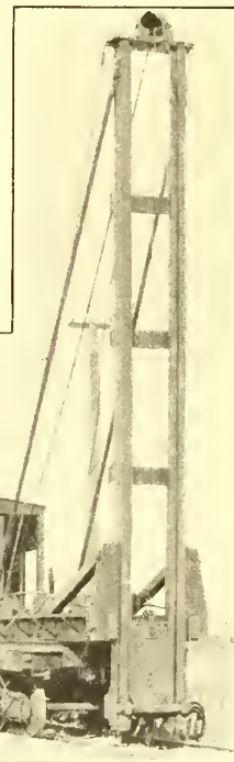
FRONT VIEW OF PILE DRIVER
