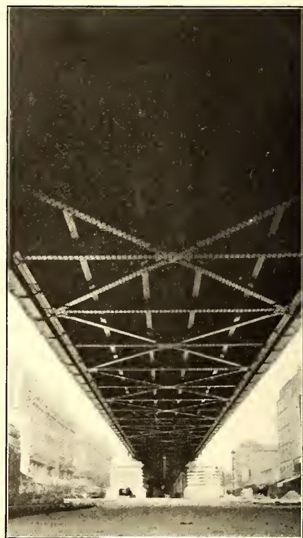
STEEL WORK ON UNDER SIDE OF VIADUCT
