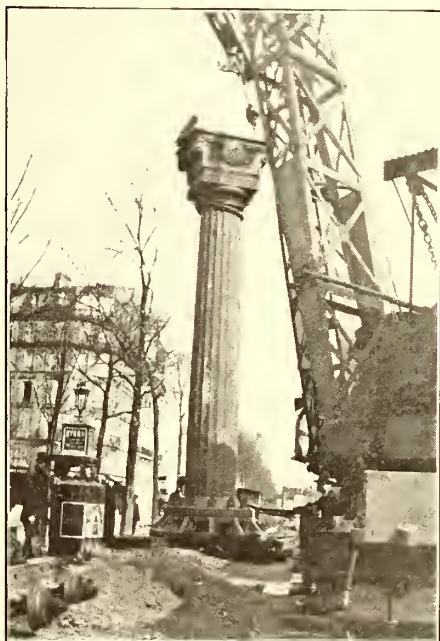
RAISING A CAST IRON COLUMN
