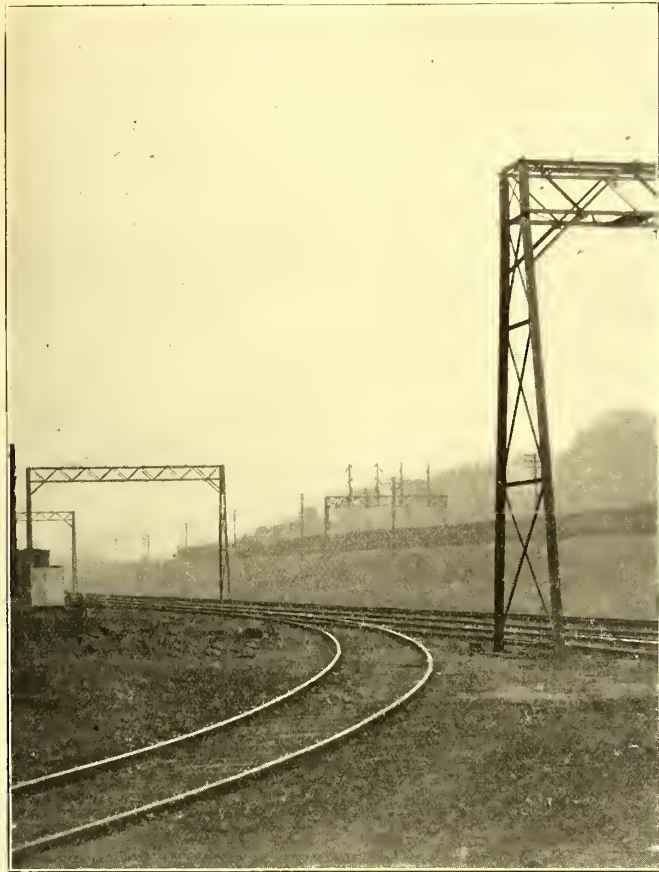
FIG. 11.—DOUBLE CATENARY BRIDGE CONSTRUCTION
