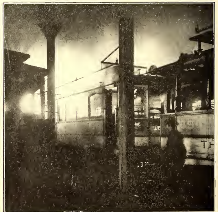
DURING FIFTH AND LAST FIRE, TAKEN AFTER REKINDLING OF FIRE AFTER IT HAD BEEN CONTROLLED BY ONE AISLE SPRINKLER
