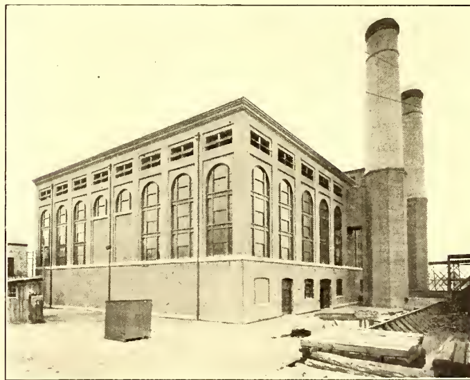
QUINCY POINT GENERATING AND SUB-STATION
