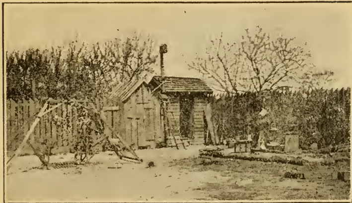
Figure 6: If these outdoor toilets must exist, they should, in all decency, be hidden from view by vines or shrubs, preferably evergreen.
