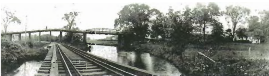
On the Waterbury extension near Cheshire Street station.
