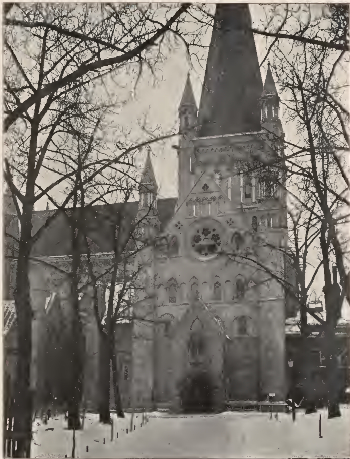
Kirken seet fra nord. The Cathedral from the north. — Die nördliche Façade des Domes.
