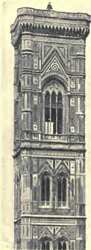
FIG. 159.—UPPER PART OF CAMPANILE, FLORENCE.
