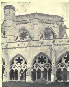
FIG. 137.—CLOISTERS, SALISBURY CATHEDRAL (SHOWING UPPER PART OF CHAPTER-HOUSE).
