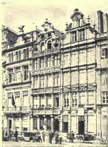
FIG. 197.—RENAISSANCE HOUSES, BRUSSELS.
