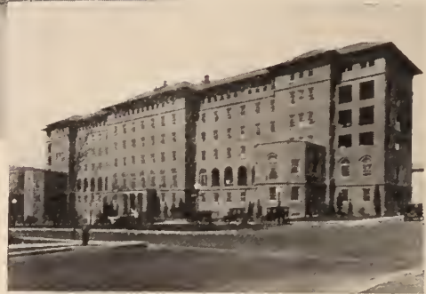
The New Union Memorial Hospital, Baltimore, Md.
