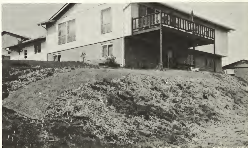
Jute netting and straw cover a newly seeded slope. Retouching became necessary when bare spots appeared in this recently established lawn.
