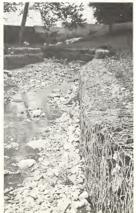
Silt laden runoff collects in this debris basin below a large site being graded for a shopping mall. As water rises in and around the metal box (above) sediment drops out, dries up, and accumulates for future use. Gabions (below) line the banks of a creek below Wilde Lake Dam. The tightly packed rocks and wire netting might be mistaken for real walls from a distance.
