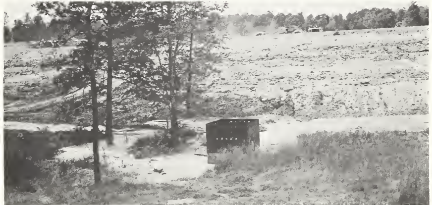
Silt laden runoff collects in this debris basin below a large site being graded for a shopping mall. As water rises in and around the metal box (above) sediment drops out, dries up, and accumulates for future use. Gabions (below) line the banks of a creek below Wilde Lake Dam. The tightly packed rocks and wire netting might be mistaken for real walls from a distance.
