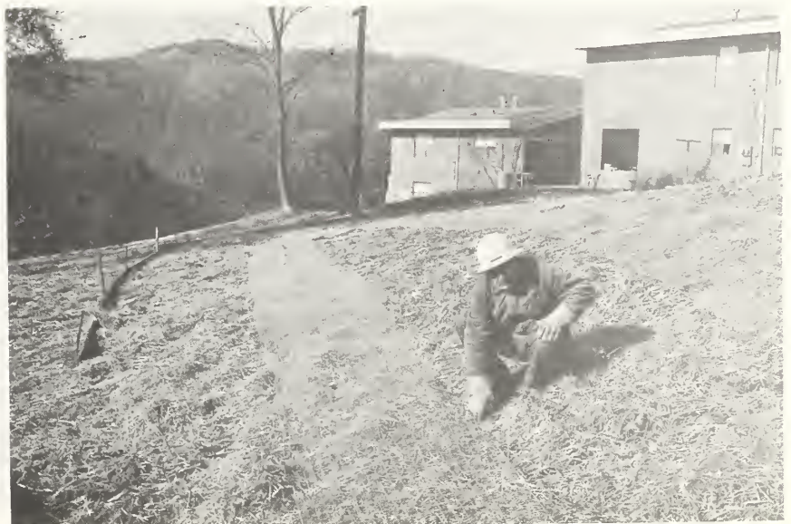
Francis Kolz, district crew member (left), and Moses Taylor, SCS soil conservationist, lay netting over a critical area seeded and mulched in November 1968. Below, Kolz looks over a finished job consisting of straw mulch, Bemis netting, and 2 by 4 planks set into a steep slope.
