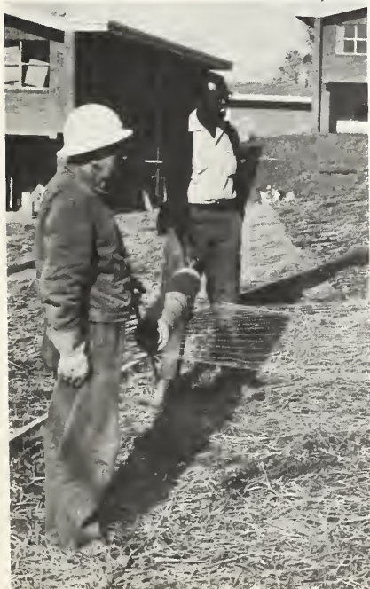
Francis Kolz, district crew member (left), and Moses Taylor, SCS soil conservationist, lay netting over a critical area seeded and mulched in November 1968. Below, Kolz looks over a finished job consisting of straw mulch, Bemis netting, and 2 by 4 planks set into a steep slope.
