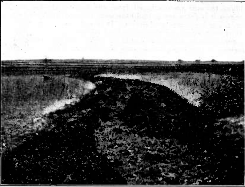
FIGURE 18.—One method of starting the construction of a terrace with the single-blade terracing machine shown in Figure 15. One round with the machine has been made, the furrows being about 8 feet apart
