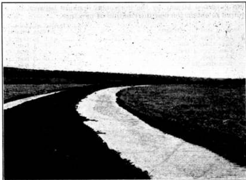
FIGURE 10.—Water standing above a circular level terrace with no outlet, after a heavy rain
