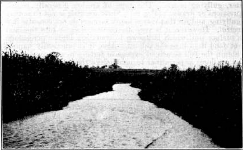
FIGURE 3.—Drainage ditch partly filled with sand washed from eroding hills
