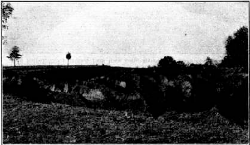
FIGURE 5.—Erosion on very silty soils which practically ruins broad areas of fertile land. Alternate freezing and thawing hasten the rate of erosion over such areas, particularly in the South
