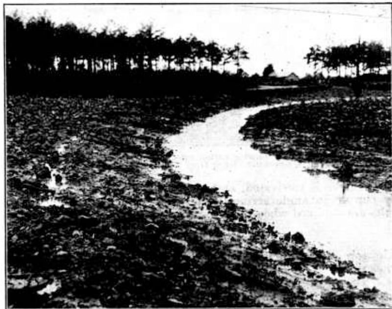
FIGURE 8.—Water flowing off at a low velocity in a broad, shallow channel of a Mangum terrace
