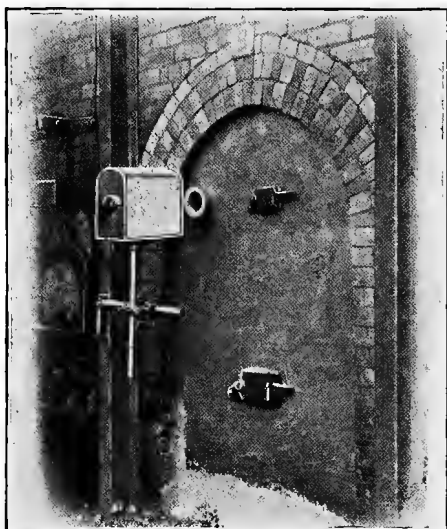
FIG. 86.—Optical Pyrometer in Position.
