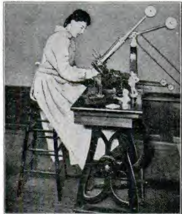
Statue-Copying Machine in Operation.
