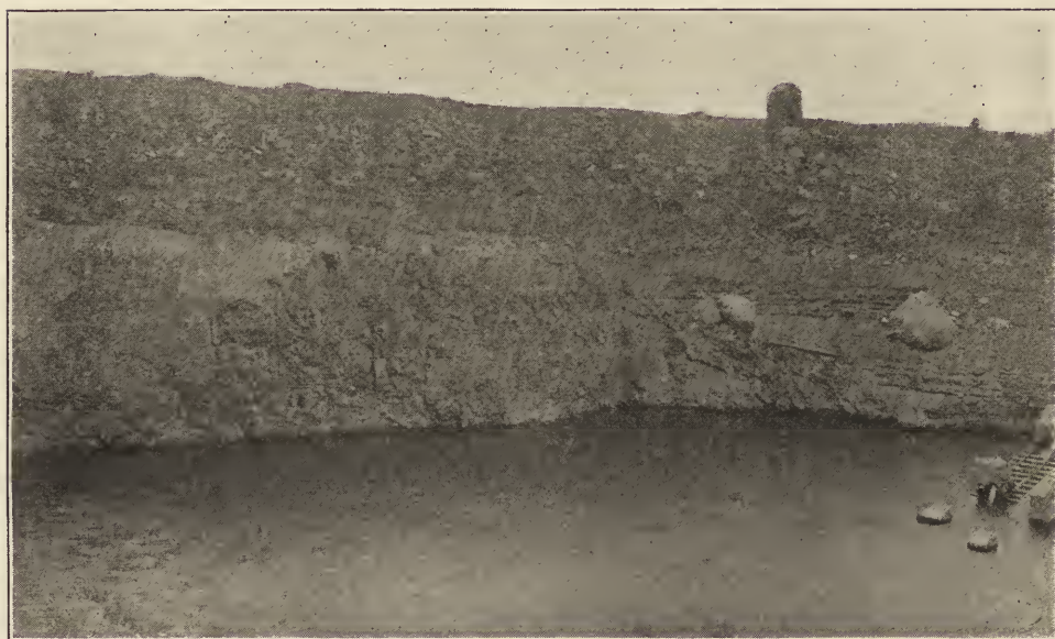
CUT FOR THE LOCK AROUND THE CASCADES OF THE COLUMBIA RIVER
