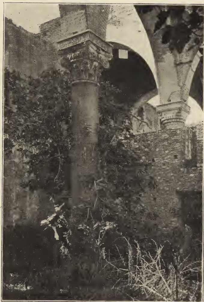
GRANITE SHAFT AND ANTIQUE CAPITAL IN THE MOSQUE [FIG. 4 OF FIRST ARTICLE]
