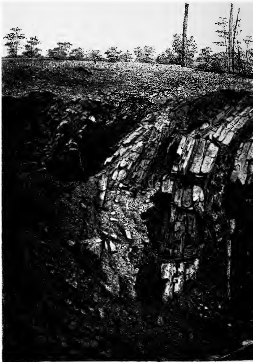
EXAMPLE OF SURFACE CREEP A on the East Broad Top Rail
