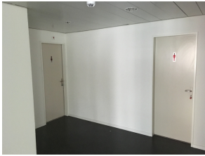
Washrooms, accesible from the separted entrace room
