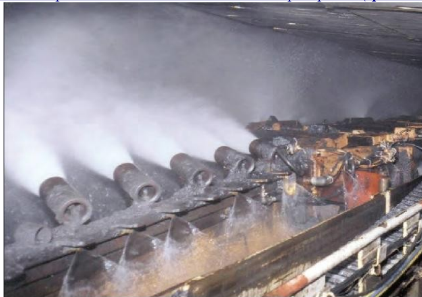
Figure 3-8.—Venturi sprays mounted on headgate splitter arm.
