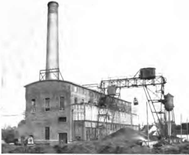
FIG. 200. View of the Power House Shown in Fig. 199.
