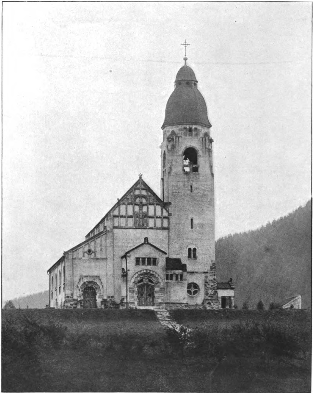
189. Kamil Hilbert. Štechovice Church.
