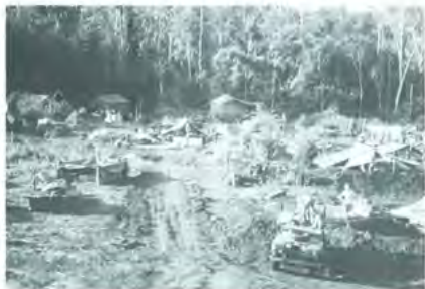
LIVING QUARTERS AT AN AUSTRALIAN FIRE SUPPORT BASE
