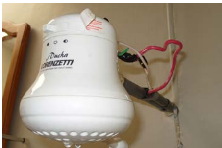
Figure 20.41 On-demand electric hot water heater. Heat is supplied to water only when needed. (credit: avidavid, Flickr)
