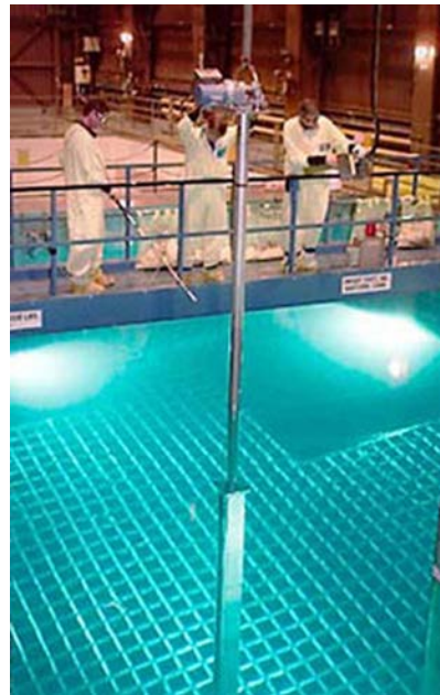
Figure 14.32 Radioactive spent-fuel pool at a nuclear power plant. Spent fuel stays hot for a long time. (credit: U.S. Department of Energy)
