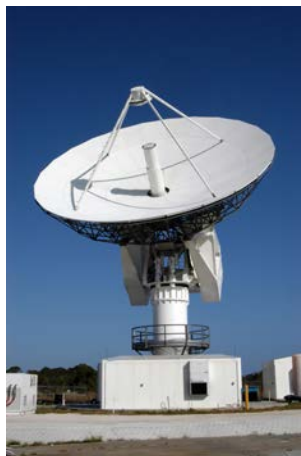
Figure 24.2 The electromagnetic waves sent and received by this 50-foot radar dish antenna at Kennedy Space Center in Florida are not visible, but help track expendable launch vehicles with high-definition imagery. The first use of this C-band radar dish was for the launch of the Atlas V rocket sending the New Horizons probe toward Pluto. (credit: NASA)
