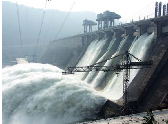
Figure 7.38 Hydroelectric facility (credit: Denis Belevich, Wikimedia Commons)
