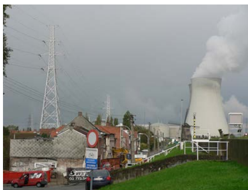
Figure 32.24 The people living near this nuclear power plant have no measurable exposure to radiation that is traceable to the plant. About 16% of the world's electrical power is generated by controlled nuclear fission in such plants. The cooling towers are the most prominent features but are not unique to nuclear power. The reactor is in the small domed building to the left of the towers. (credit: Kalmthouts)
