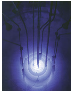
Figure 17.39 The blue glow in this research reactor pool is Cerenkov radiation caused by subatomic particles traveling faster than the speed of light in water. (credit: U.S. Nuclear Regulatory Commission)
