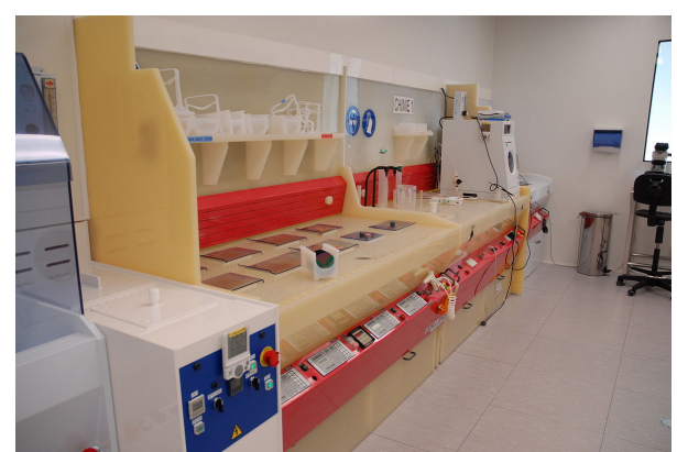
Etching tanks used to perform Piranha, Hydrofluoric acid or RCA clean on 4-inch wafer batches at LAAS technological facility in Toulouse, France
