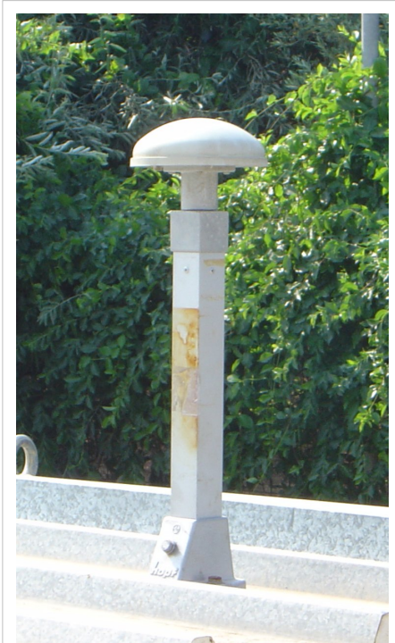
This antenna is mounted on the roof of a hut containing a scientific experiment needing precise timing.
