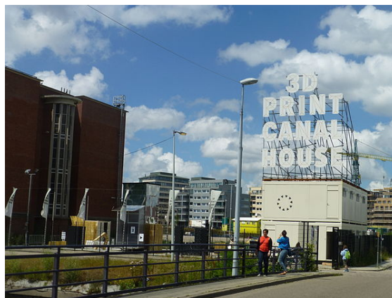
Printing 3D house project at Amsterdam
